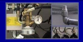
system that protects the data center equipment and a 'wet' or 'pre-action' sprinkler system that is used to save the building. Also, fire detectors and alarm system will warn the people.
