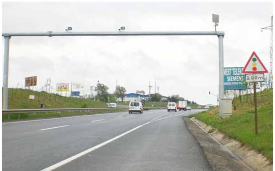
Traffic management in Corlu
